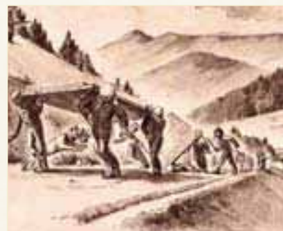
La construction des baraques-1941 Bau der Baracken-1941 Construction of the prison huts-1941
